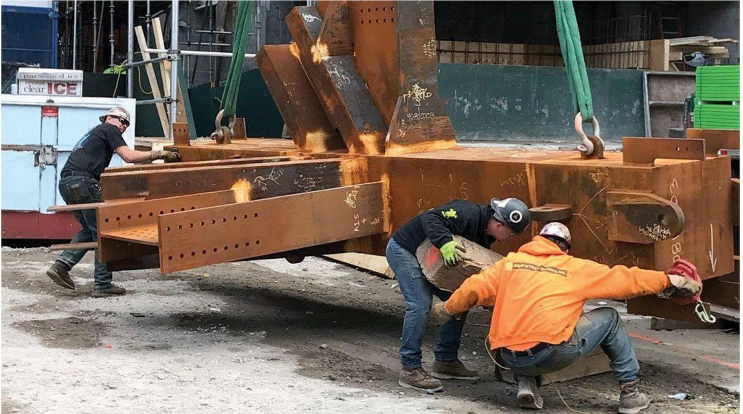
**CAST CONNEX**—A team makes preparations for a High Integrity Block node lift. These Cast Connex blocks are specially engineered and manufactured solid steel elements which simplify the making of heavily loaded structural connections and elements.
