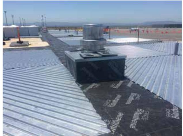
Figure 4. Shell infill – to the left is the installation of light gauge framing; it supports the metal decking shown on the right, creating a level roof plane. Courtesy of MVVA Architects.
