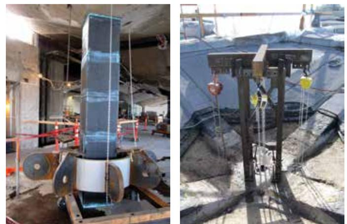
Figure 3. Olson's lifting rig – to the left is a casting being lifted into place; the rig is on the right. Note the top of the roof ribs.
